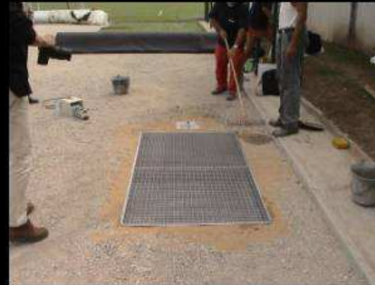
Adjustment of the ground draining support
