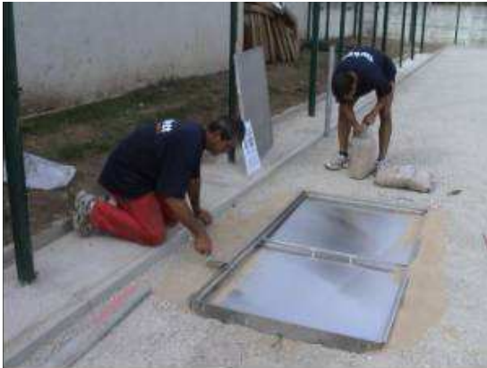
Installation of the water collecting unit
