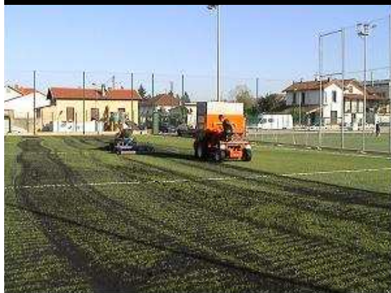
Spreading and brushing SBR all over the field
