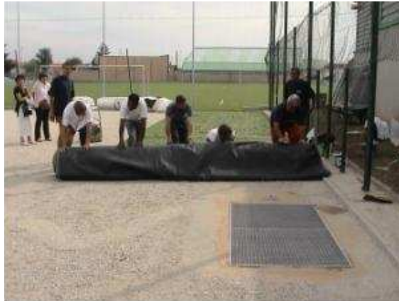
Unfolding of a roll of synthetic turf
