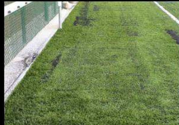
Discharge of SBR to the top of the water collecting unit
